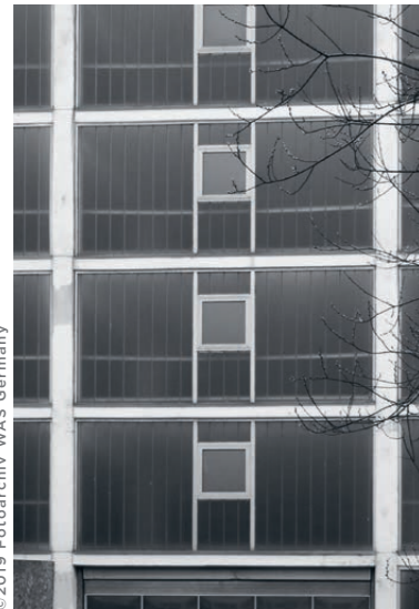
The six-storey new warehouse covering a total of 5,000 m 2
